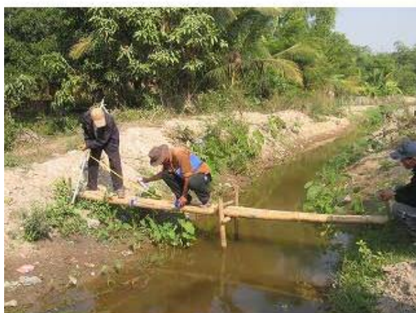
Making Cross Section Area at Bamboo Bridge at Tertiary Canal
