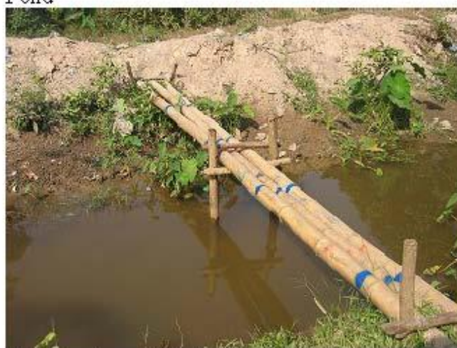
Construction of Bamboo Bridge for all Measurement Points
