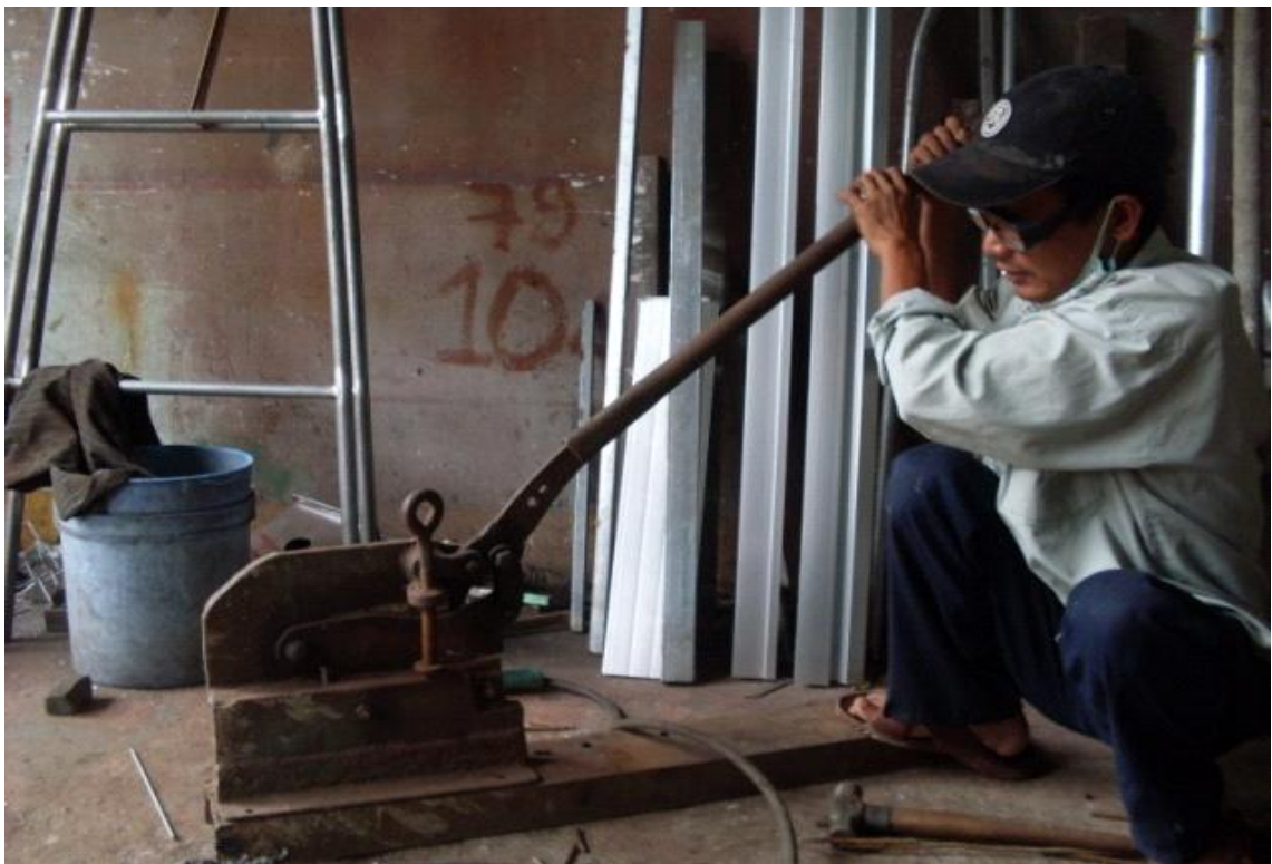
Figure 40 Select metal, welded frame in shape, Cutting iron
