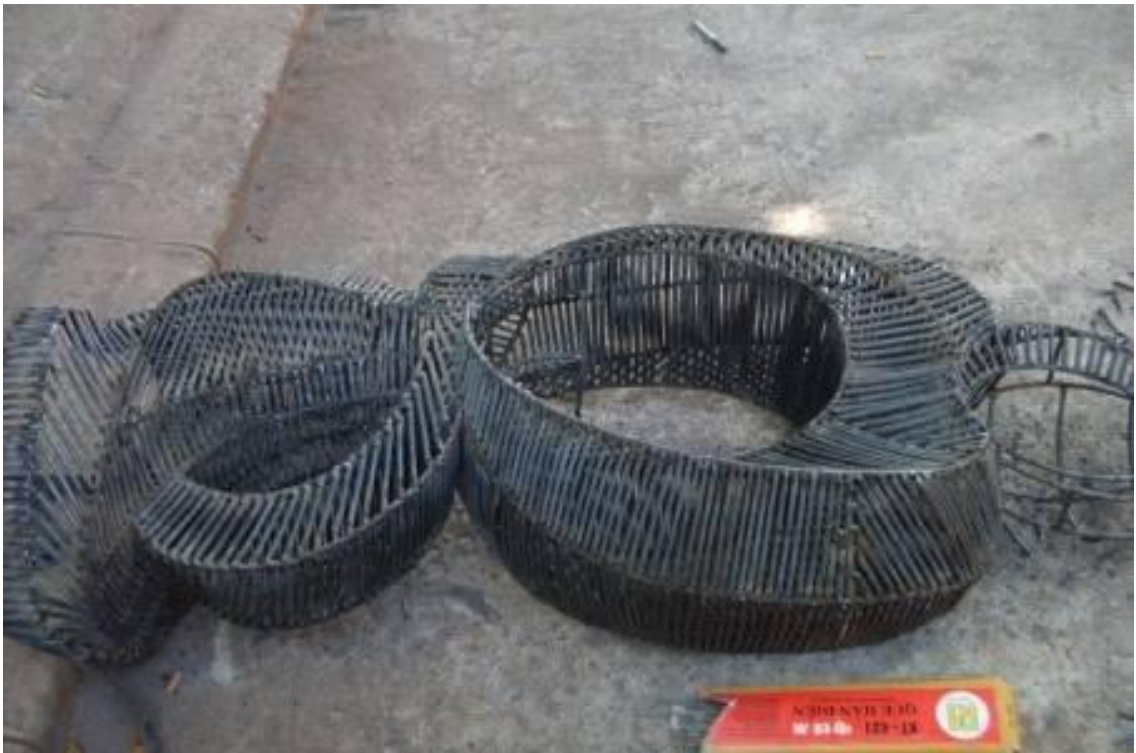
Figure 47 Weld details, Cleaning work
