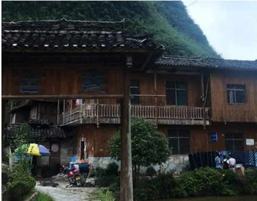
Figures 6 ‘Ganlan,’ the name of Bouyei architecture. The hanging mountain roof extends beyond the gable wall and is suitable for the mild and rainy southern climate. Source: Kong Ruoyue, accessed 2015
