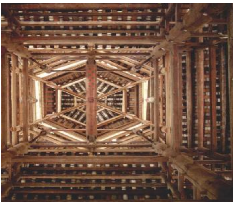
Figure 44 The internal structure of the Drum Tower
