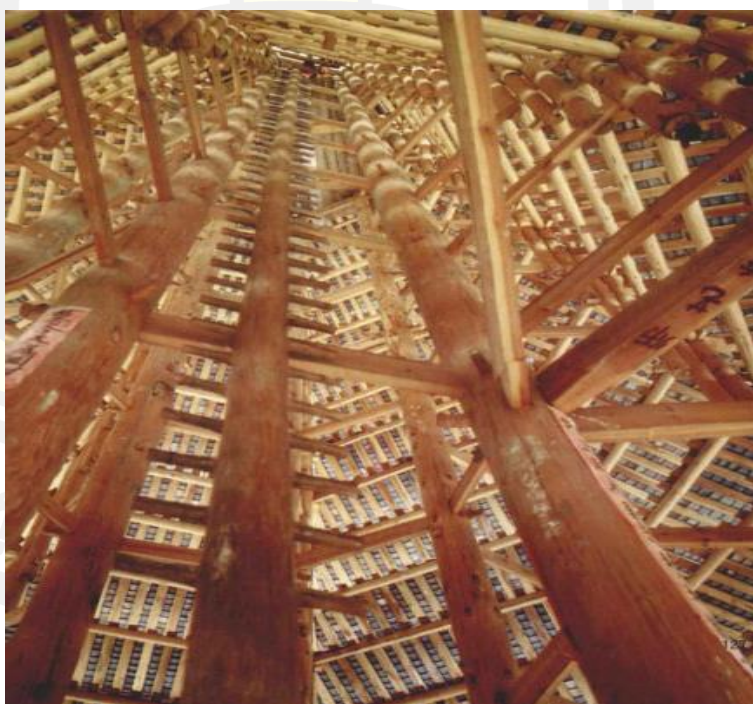
Figure 45 The internal structure of the Drum Tower
