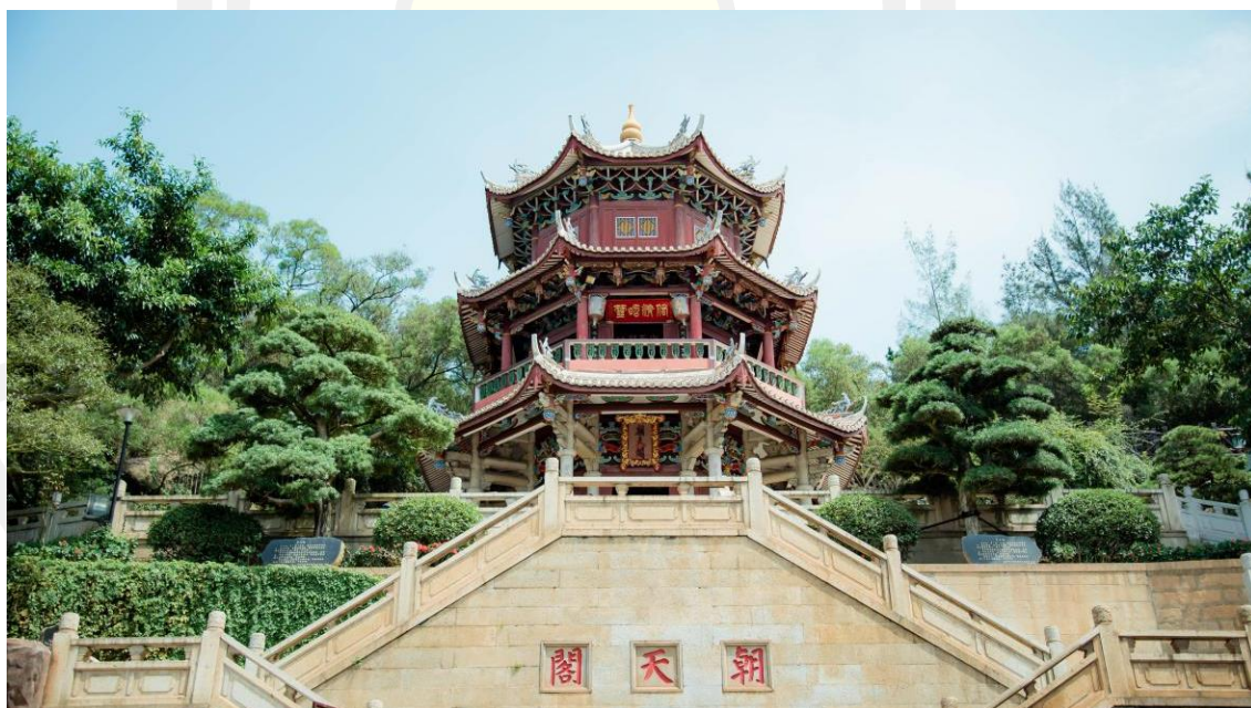
Figure 20 The Chaotian tower Source: Photographed by Ke Yihan, 2020
