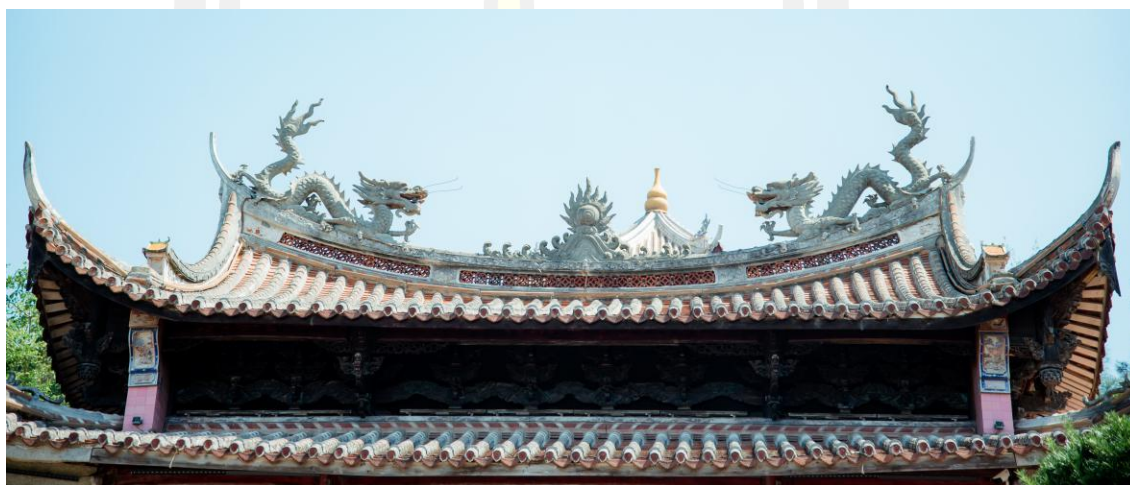
Figure 24 The dragon statue on the ridge of the roof
