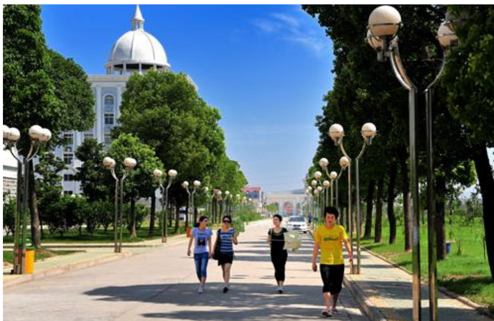
Figures 44 Jingzhou Vocational and Technical College Teaching Building by Wu Peng (2015)
