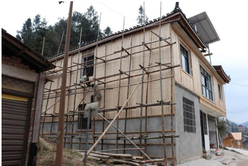
Figure 4. 19 Houses under repair in Zaidang Dong village
