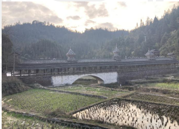
Figure 4. 3 The "Fengyu Bridge" across the mountains
