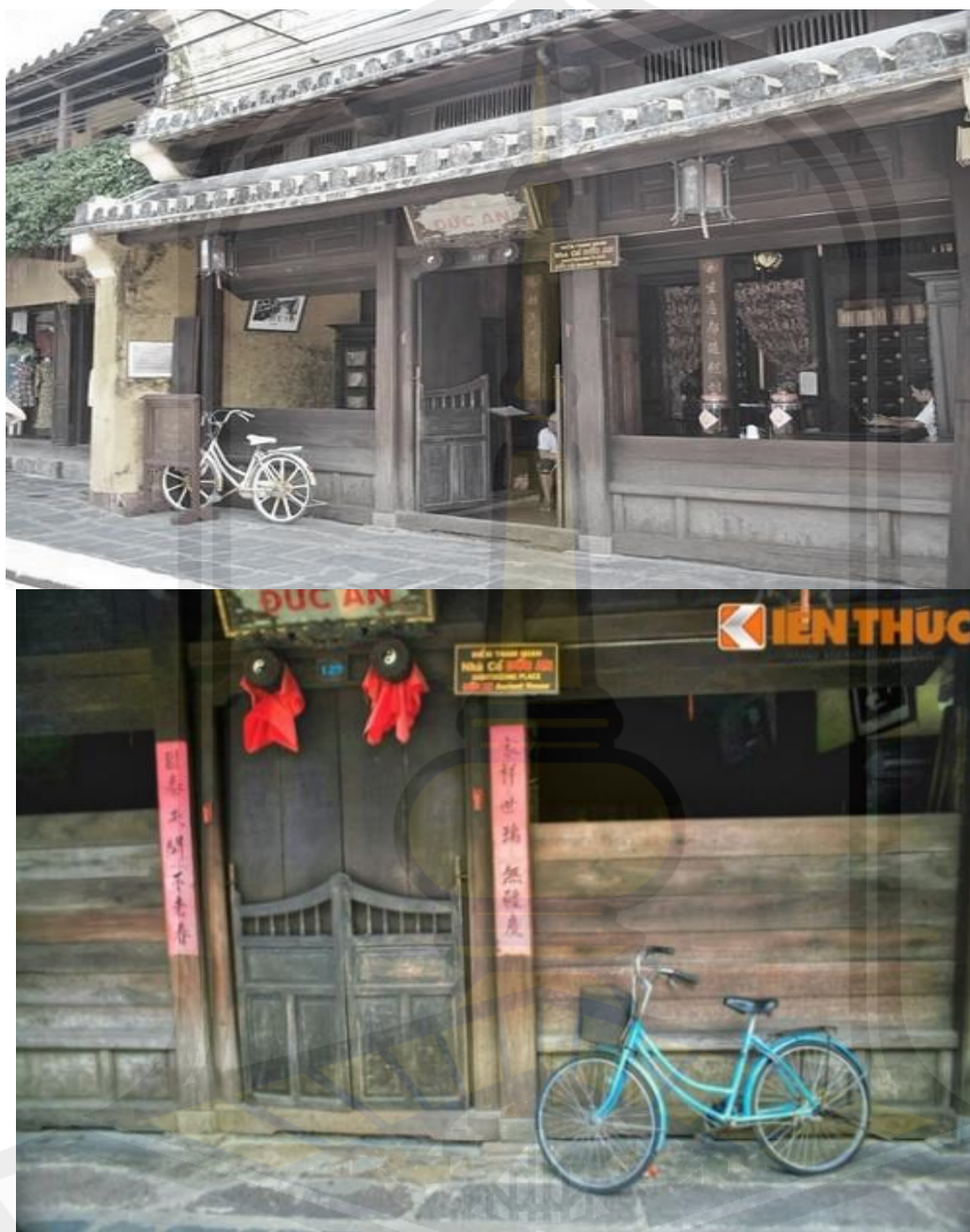
Figure 50 The special door of the house. Source: internet
